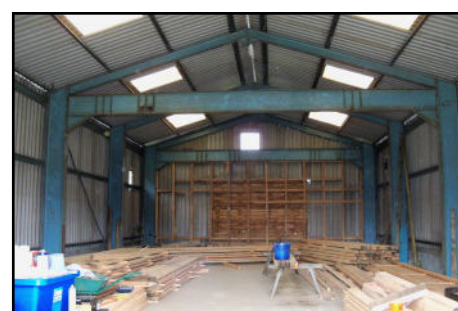
Interior of barn showing timber and planks ready for hand finishing
